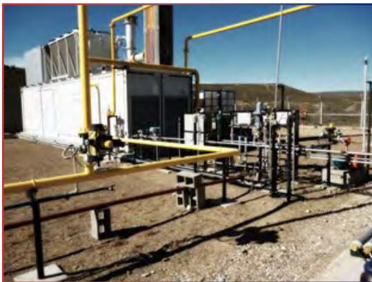
Electrolysers at the Hychico plant. Image source: Hychico SA
